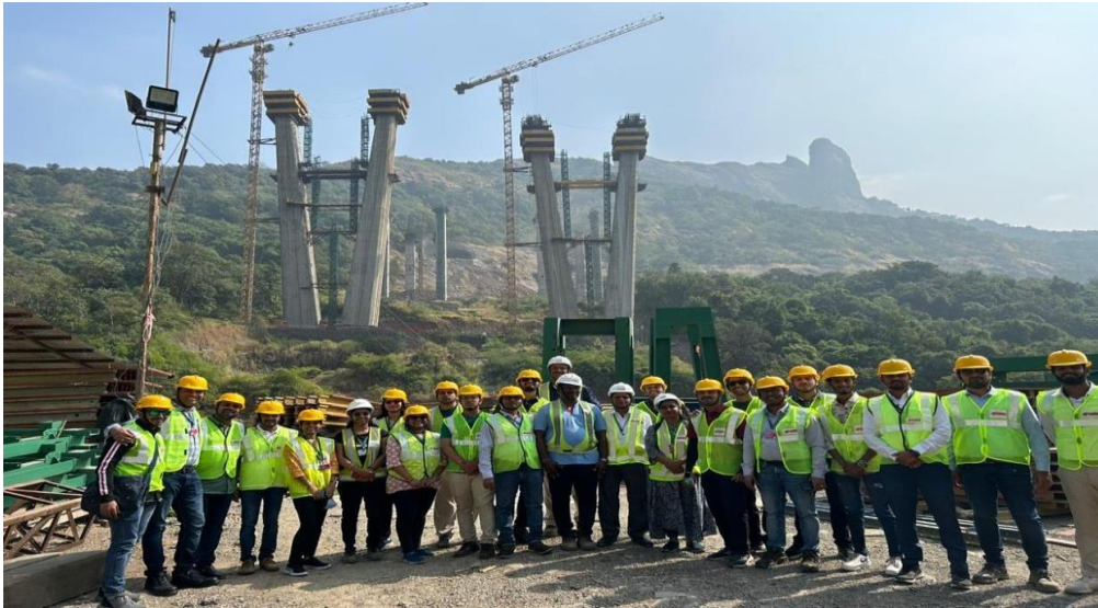
At the viaduct site
