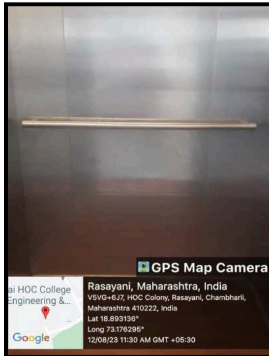
Figure : Handrails in Lift1 for disabled
