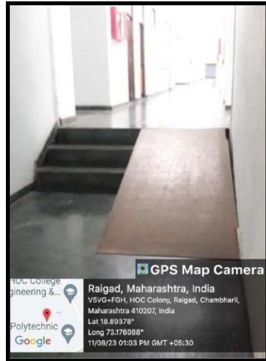
Figure 4: Ramp near re recreation area
